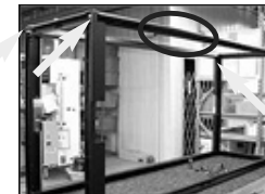
Ensure Clips on Vertical Frames Face Out
