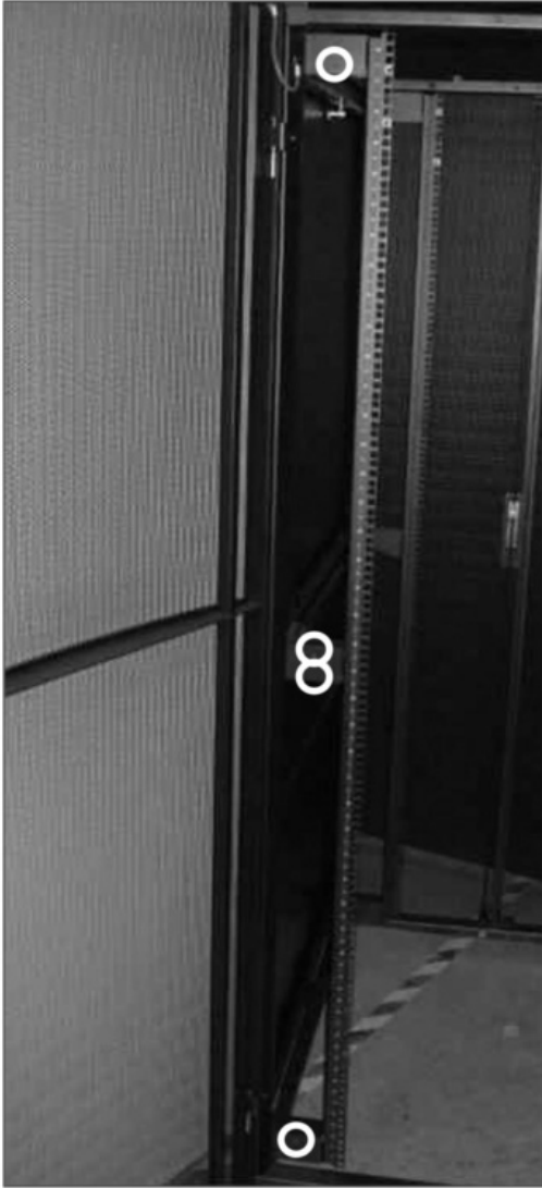
ZERO-U PANEL MOUNTING HOLE LOCATIONS
