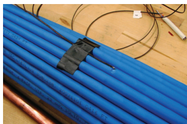
Photo 2. Placement of temperature sensing Thermocouple
