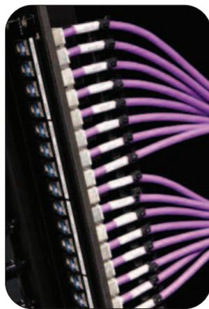
modern data centre ease of maintenance is important in order to rectify any issues that may arise. The University's data centre design means that, for example, individual ports rather than the entire panel can be changed if and when required and access to the racks is made as simple as possible.'
