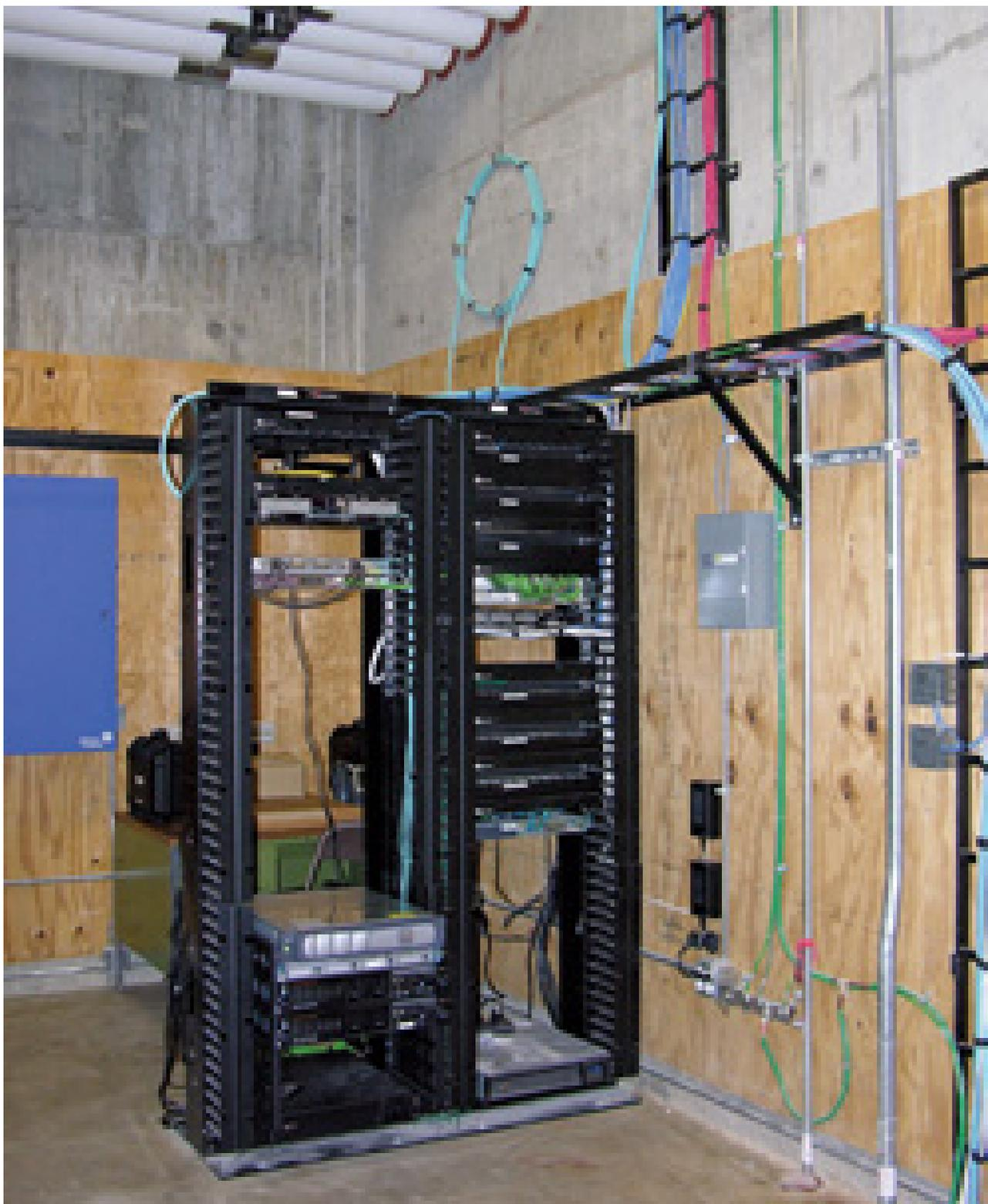
The museum established a high-availability location, shown here, in the new East Building. The location is tied to a separate backup generator and replicates the entire hosted environment via 10-Gbit/sec fiber connections. If the primary data center and generator are lost, the high-availability location can keep the museum 100-percent online.
