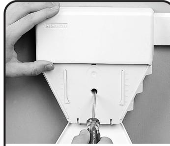
**11** Using a philips or flathead screwdriver tighten the captive screw located under the hinged label cover.
