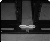
Make sure both cabinets that the VPC will be installed between, are level and properly bayed together using all (4) baying brackets. See Baying Instructions.
