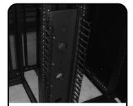
Install the (2) cable management fingers to each side of the VPC using the (4) Phillips screws and washers as shown.
