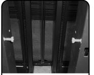
Install the (4) shoulder bolts provided onto the inside of the VPOD Frame as shown, using the 5/32" Allen Tool. The VPC may be mounted in the top half or bottom half of space between bayed cabinets.
