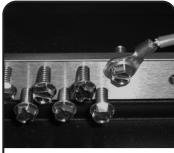
To bond the cabinet to the Ground Bar, install one preterminated end of the 18" #10 wire to the ground bar using one of the 12-24 screws provided.
