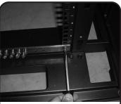
Using the (2) 12-24 x 5/8" thread forming screws, attach the ground bar to the cabinet.
