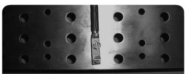
Remove any oxidation, etc. from the mounting surfaces and apply a coating of antioxidant material. Attach the opposite end of the 96" ground wire used above to the main ground bar or to an extension of the main ground bar.
