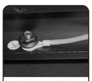
Attach other end of the #10 wire to the bonding post located at the middle of the lower horizontal support using the M6 flange nut provided.
