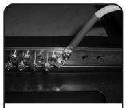
Remove any oxidation, etc. from the mounting surfaces with abrasive pad and apply a coating of antioxidant material. Using (2) of the 12-24 x 1/2" machine screws attach one end of the 96" ground wire to the ground bar.
