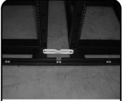
Make sure both cabinets that the Blank will be installed between, are level and properly bayed together using all (4) baying brackets. See Baying Instructions.
