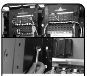
Position the vertical channel (P/N: RS-CNL or RS-CNL3) on the end of or between the RS-07 series racks. Align mounting holes and insert bolts. Install washers and nuts. Tighten nuts securely.
