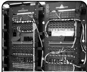
Completed RS-CNL installation showing vertical cable management.
