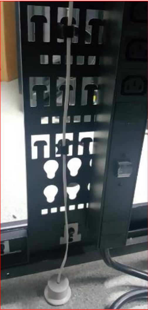
Place Sensor on the floor beneath the Cabinet
