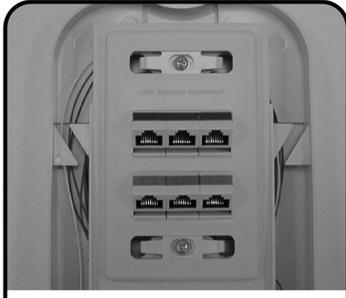
**11** Terminate and mount the outlets in the faceplate per the manufacturer's specifications and label the faceplate accordingly.
