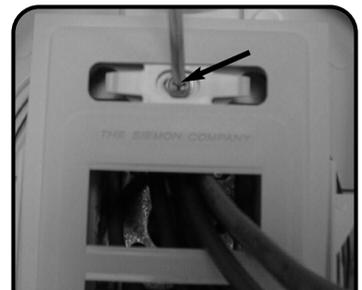
**10** Secure the Siemon CT® or MAX® series faceplate (or equivalent) onto the FOB using two of the self-tap screws provided.
