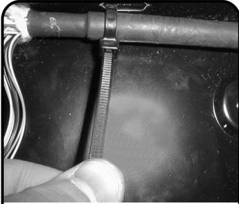
**11** Secure the cable jacket to the tray using a cable tie inserted through the lanced tab formed into the sidewall of the tray.
