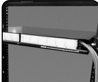
**17** Disengage latch as in Step #3 and slide tray back to the closed position.
