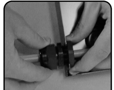
**10** If optional Compression Fitting is used – Use in place of grommet. Position the fitting at least one meter (3.28 ft) from the cut end of cable. Tighten the clamp nut against the cable jacket. Loosen the hex nut and insert the externally threaded portion of the fitting into the selected cable access hole. Re-tighten the hex nut to secure the fitting to the tray.
